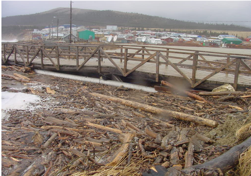
Photo 1: Damaged bridge carrying main water and sewer line, 2004.
